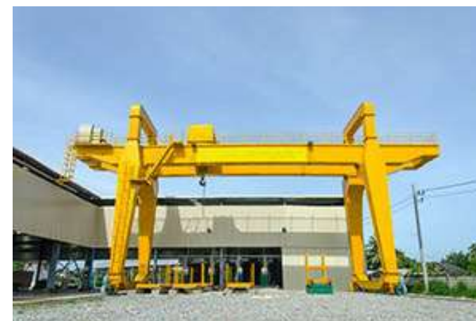
Fig.3 Image of a Gantry Crane
